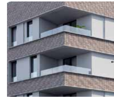
JTB Architecture Les Pavillons-sous-Bois © JTB Architecture
